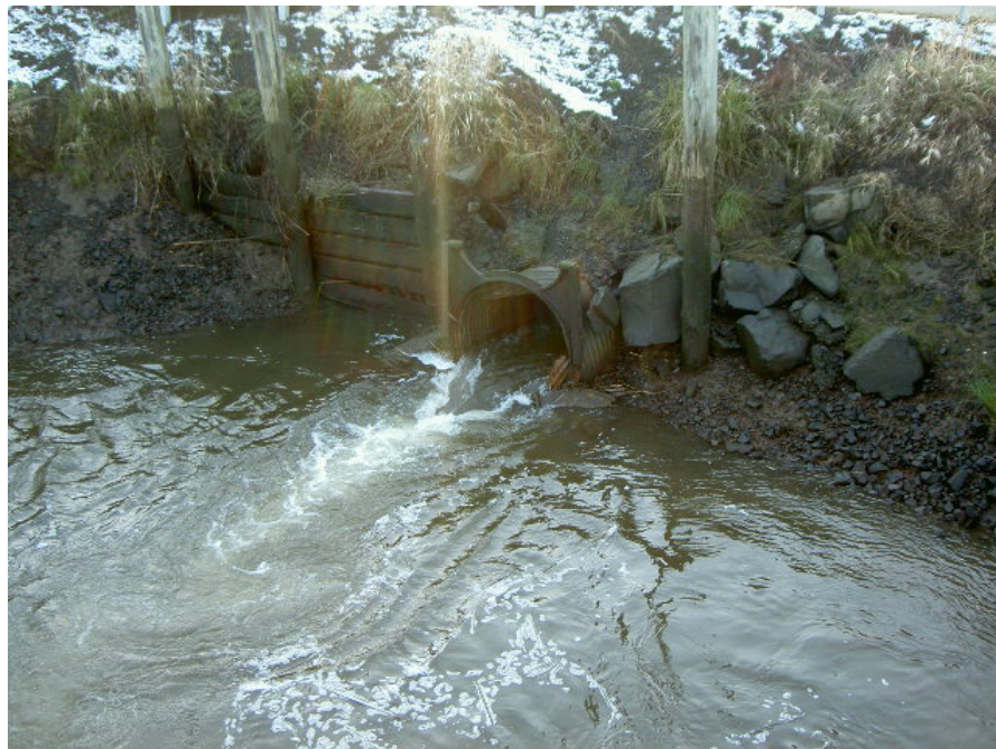
Figure 4. Pre-restoration conditions: Failing Tidegate Structure
