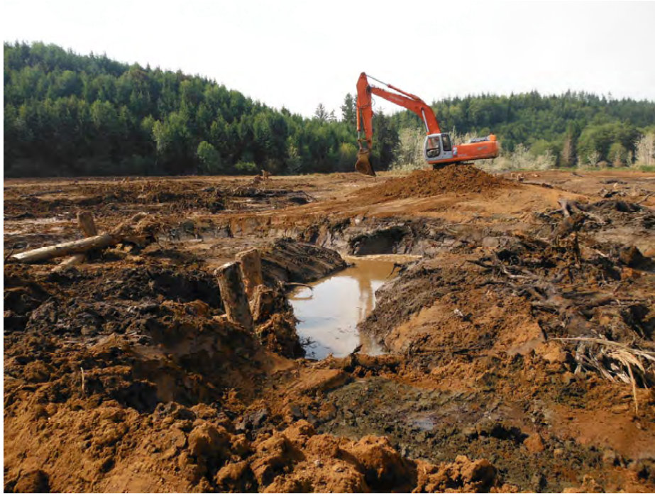
Figure 4. Excavation of New Tidal Channels at Colewort Creek
