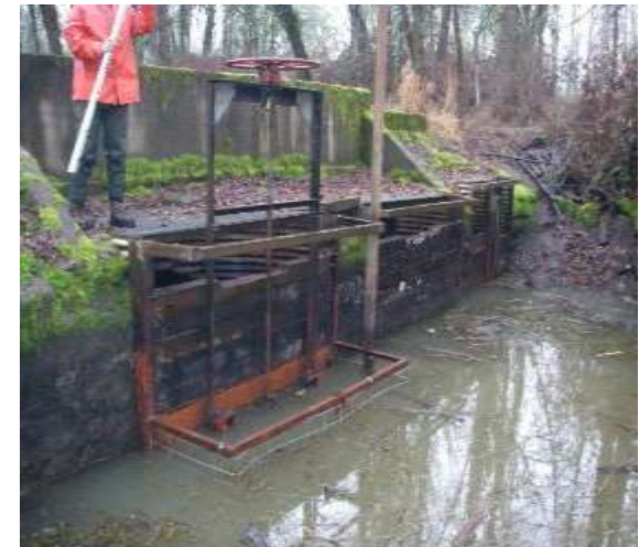
Water control structures (WCS)
