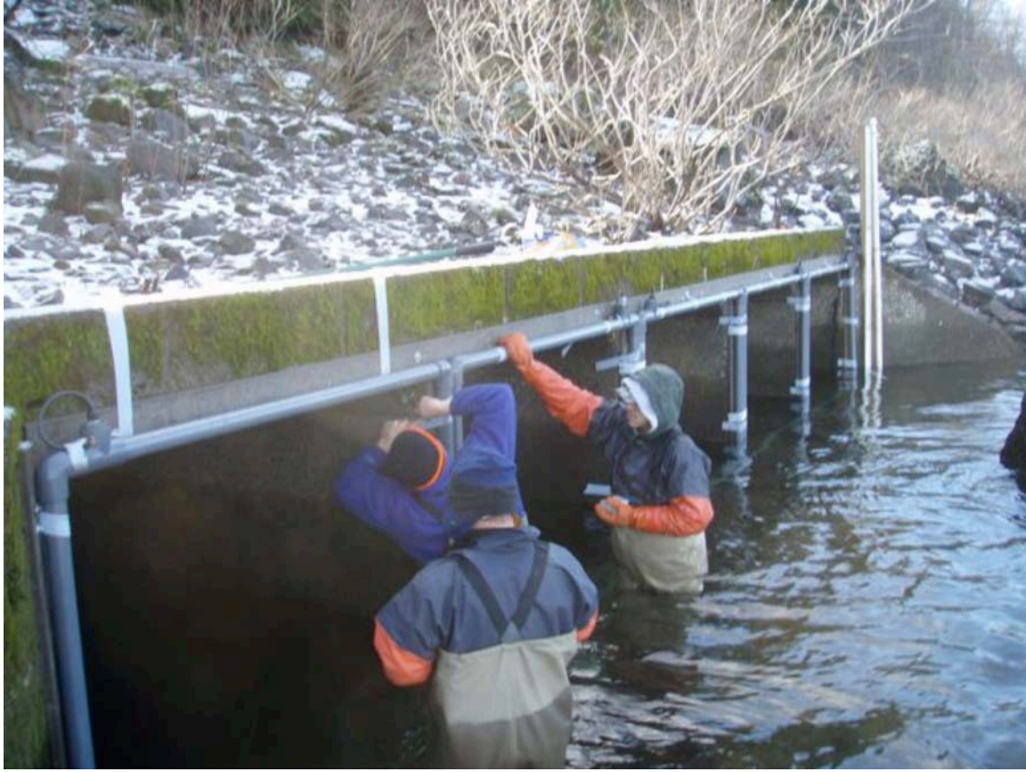
Figure 67. PIT tag array at Horsetail/Oneanta Creeks.
