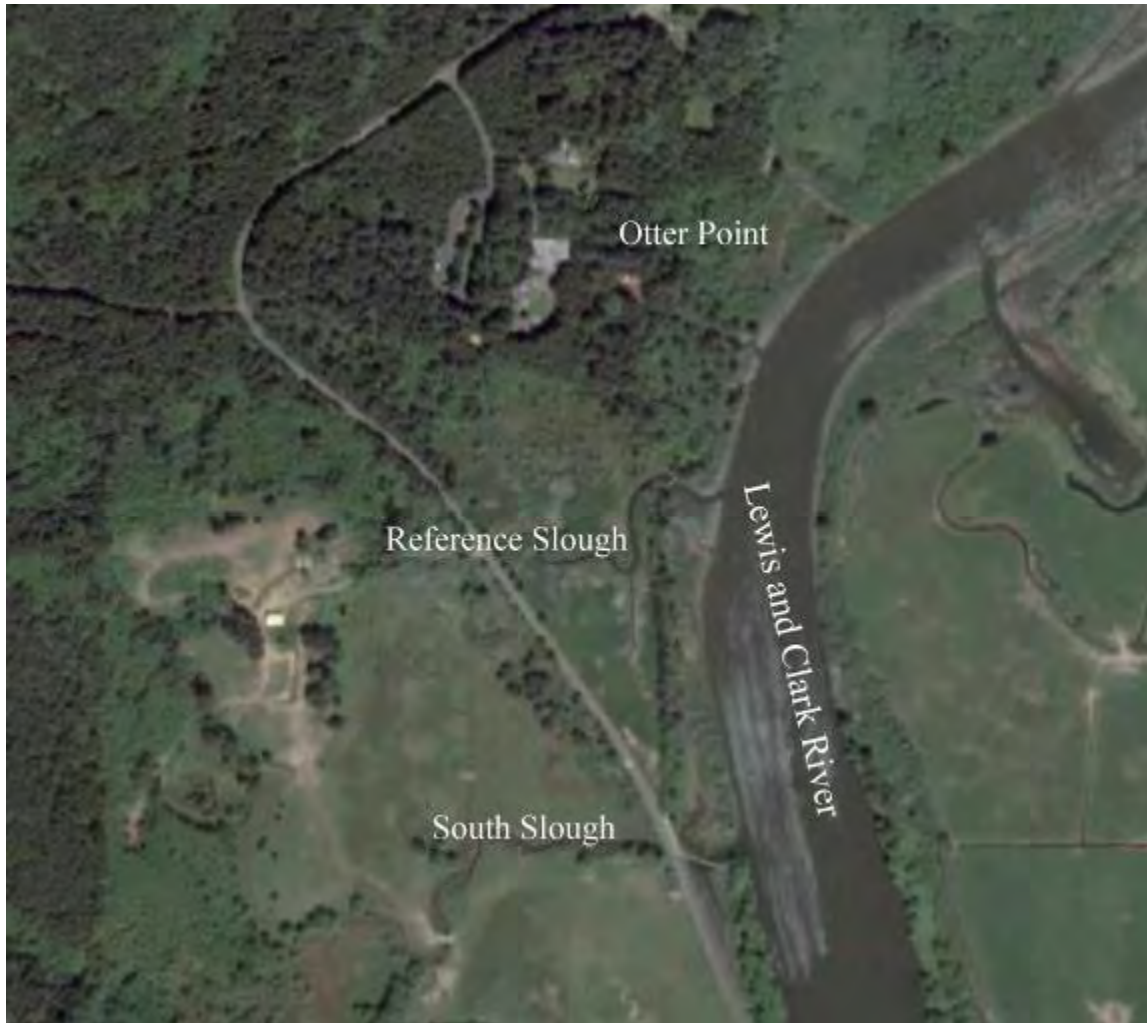
Figure 71. South Slough tidegate removal/bridge installation site, located on the Lewis and Clark River mainstem, including the nearby reference slough (Alder Creek) and current dike breach site, Otter Point.
