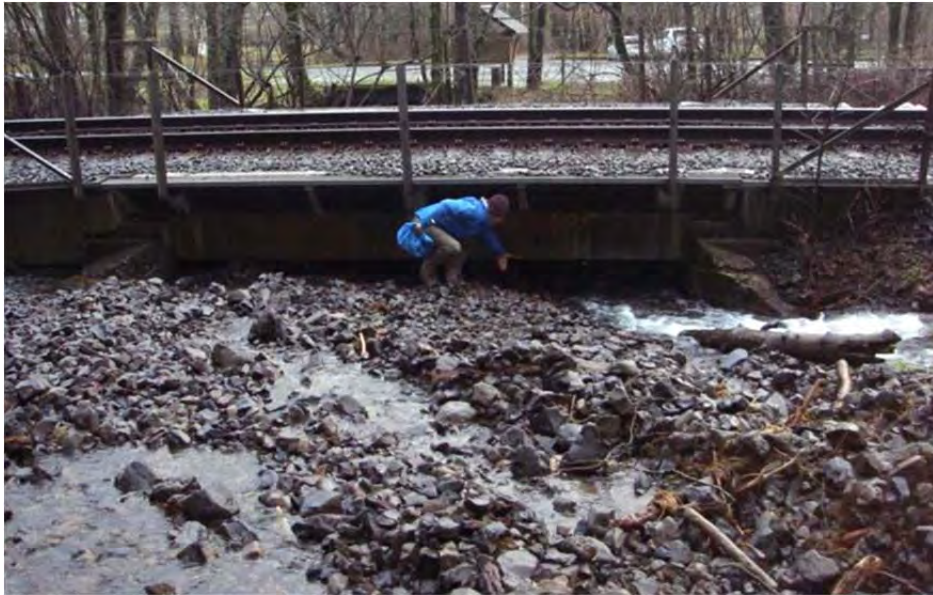
Figure 41. Wahkeena Creek railroad bridge. View is looking downstream. Note there is less than 1 foot freeboard remaining across the majority of the span.
