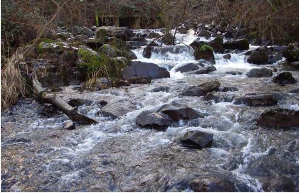
Figure 39. Roughened chute located immediately below the I-84 culvert. View is looking upstream.
