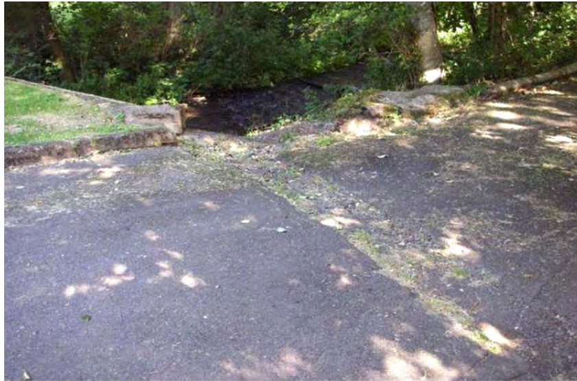
Figure 44. Benson State Recreation Area parking lot discharge to Wahkeena Creek (Reach 6). Creek can be seen in background of photo.
