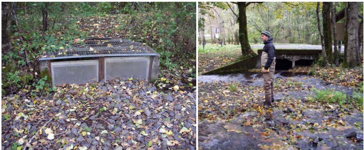
Figure 42: Hartman Pond diversion structure (left photo) and park entrance road culvert (right photo; looking downstream). Note that right barrel of culvert is partially clogged.
