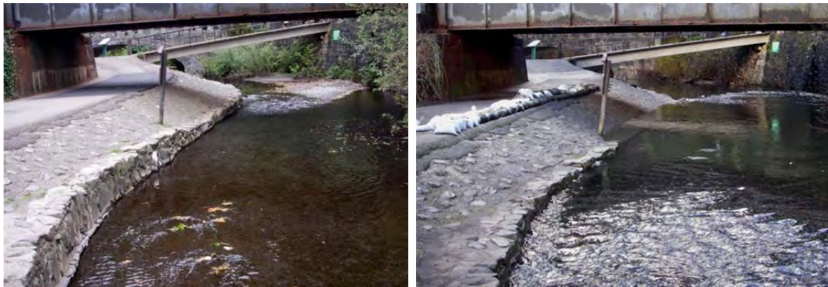
Figure 34: Multnomah Creek – Reach 1. View is looking upstream. Note loss of channel capacity between October 2010 (left photo) and February 2011 (right photo) due to aggradation during a January 2011 high flow event.
