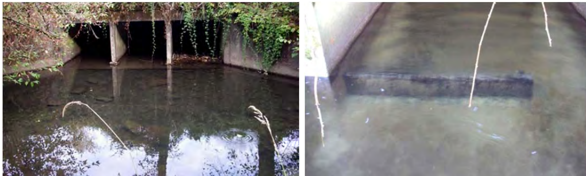
Figure 38: Confluence of Wahkeena and Multnomah Creeks & inlet to I-84 culvert (left photo) and baffles located within the three culvert barrels (right photo).
