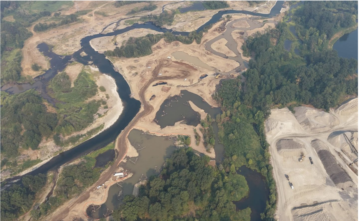
Before and construction phase photos of the Ridgefield Pits portion of the EFLR Reconnection Project site. The date of the upper photo is unknown; the lower photo is dated August 4, 2026 and was provided by Tapani.
