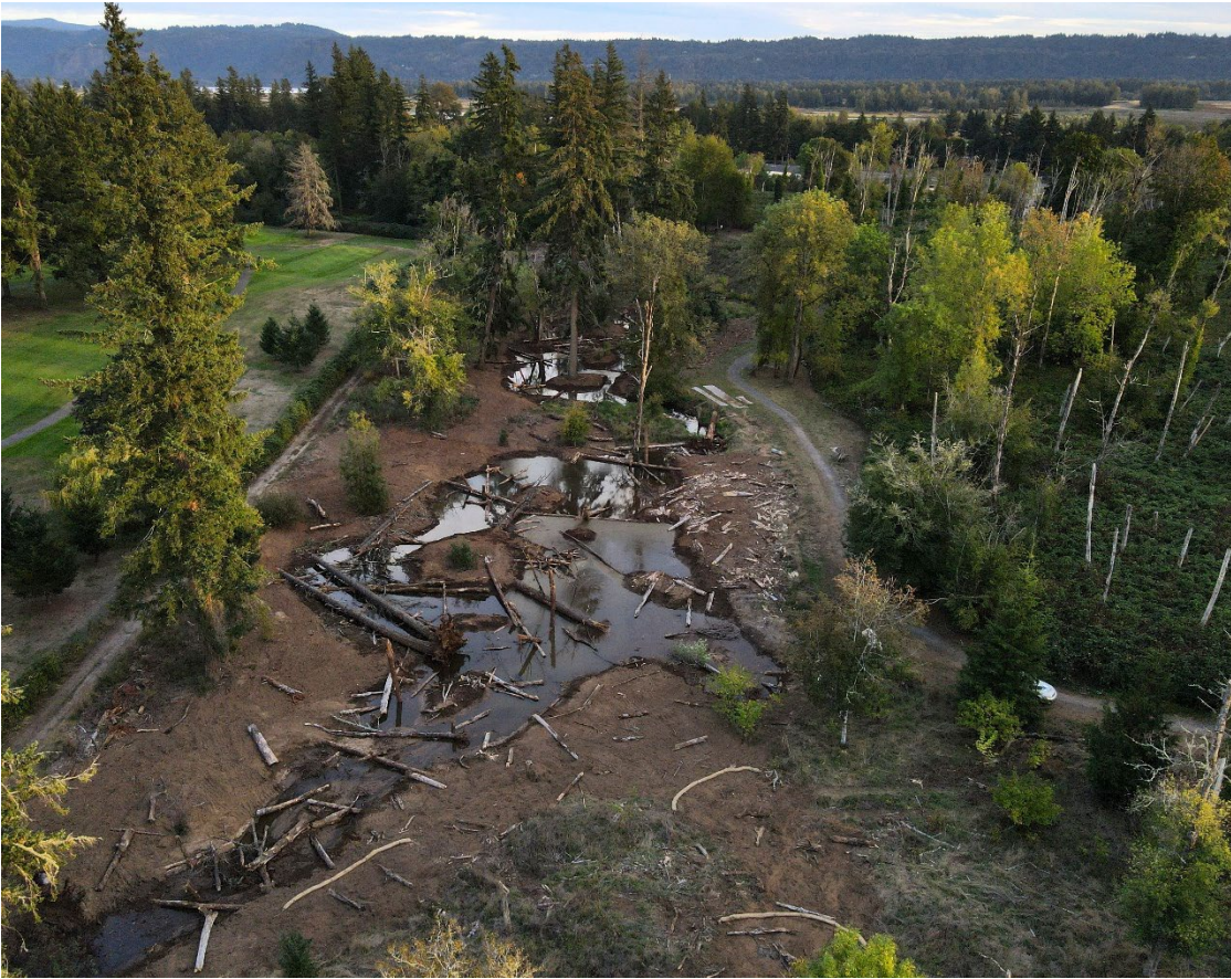
AFTER CONSTRUCTION (October 2025)
