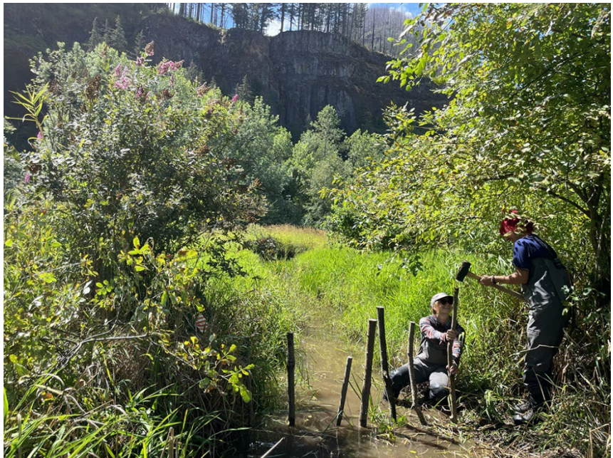
4 Pounding in stakes for a beaver dam analog
