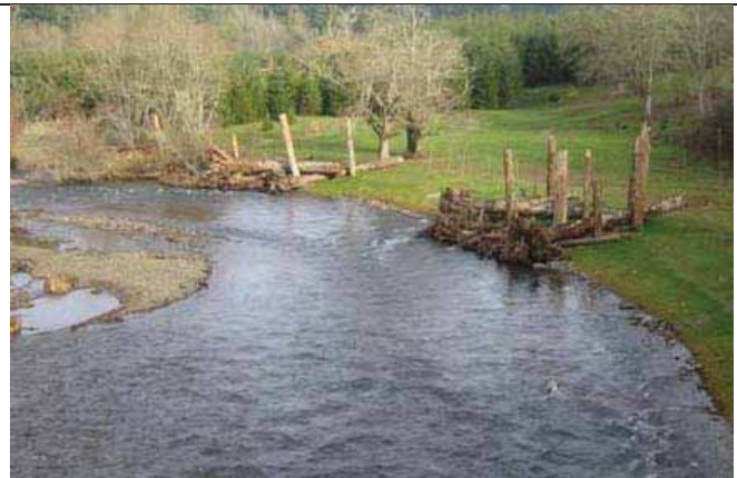
Example of Constructed Meander-bend Log Jams
