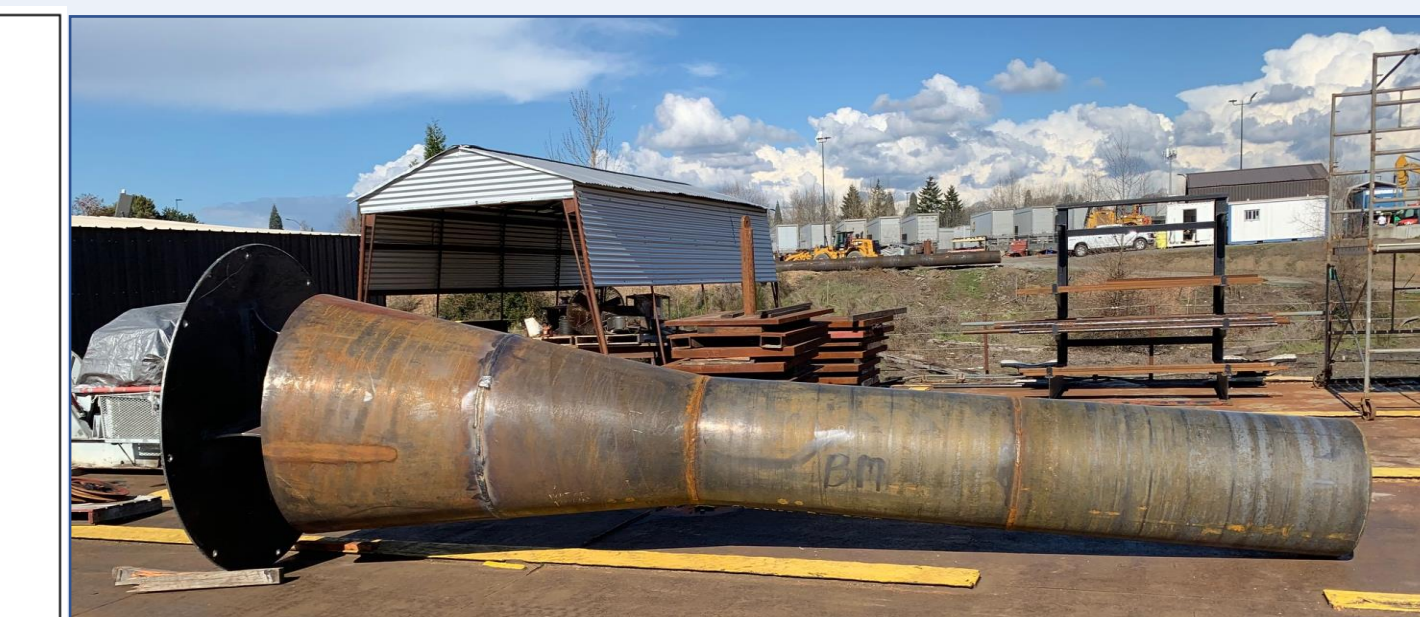
Diffuser in final stage of fabrication, MAR 2021
