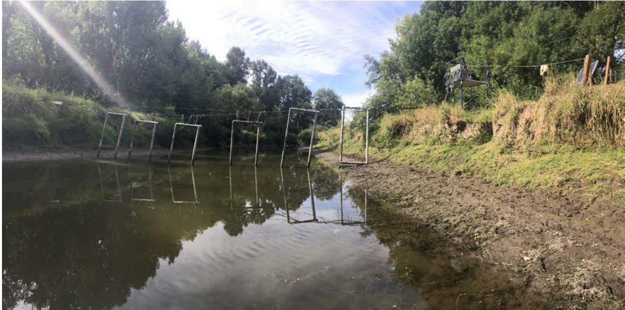
Figure 8. Image of the new PIT detection system at Campbell Slough, installed February 2018.
