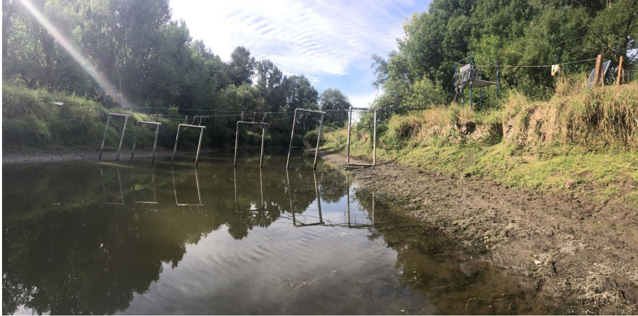
Figure 7. Image of the new PIT detection system at Campbell Slough, installed February 2018.
