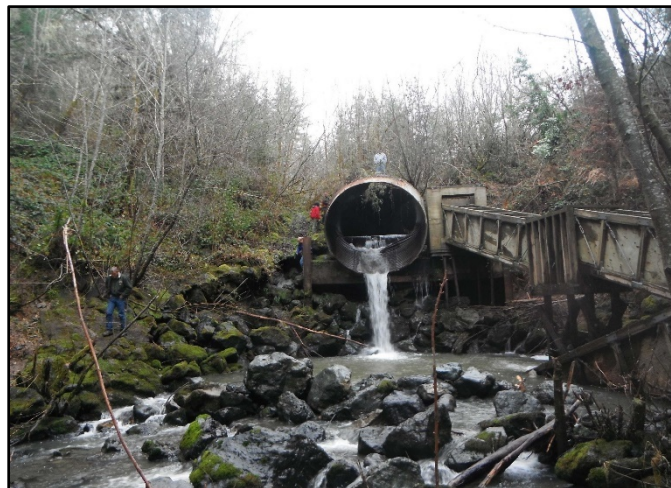
Figure 1. Pre-project photo: Large culvert perched high above stream and ineffective fishway on right.
