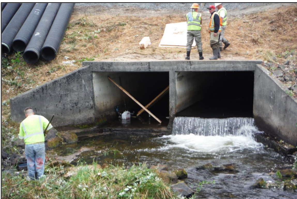
Figure 1. Pre-project photo showing how the baffle created a perched condition/waterfall on the right side of culvert.
