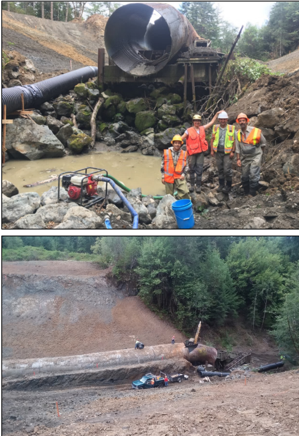
Figure 2. Project implementation photos: Fish salvage before removal of the culvert (top). Exposed culvert and slope grading during removal of the culvert (bottom).
