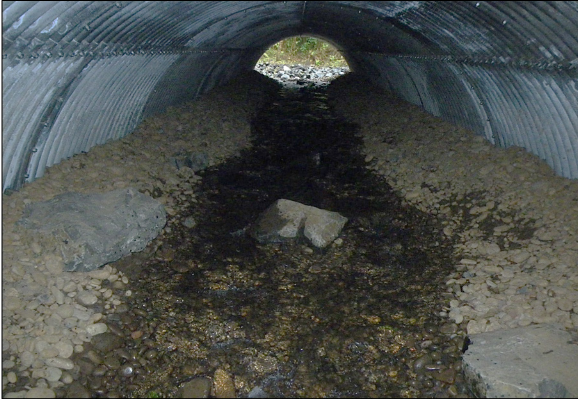
Figure 5. Completed structure has a defined low flow channel with minimum flow depths, hydraulic diversity, streambed and streambanks rebuilt inside the structure to mimic upstream and downstream conditions, and flood widths that meet or exceed 1.5 times active channel width.
