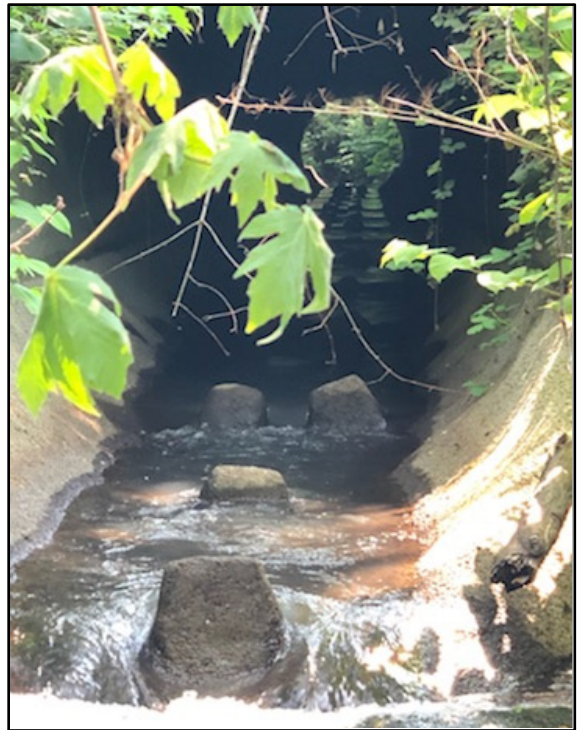
Figure 3. Pass Creek, post retrofit, showing smoothed concrete and “fish rocks” installed throughout invert of culvert to provide localized velocity reduction (left). Another example of “fish rocks” is shown (right) from a separate project, as the Pass Creek fish rocks were somewhat undersized for expected velocities.
