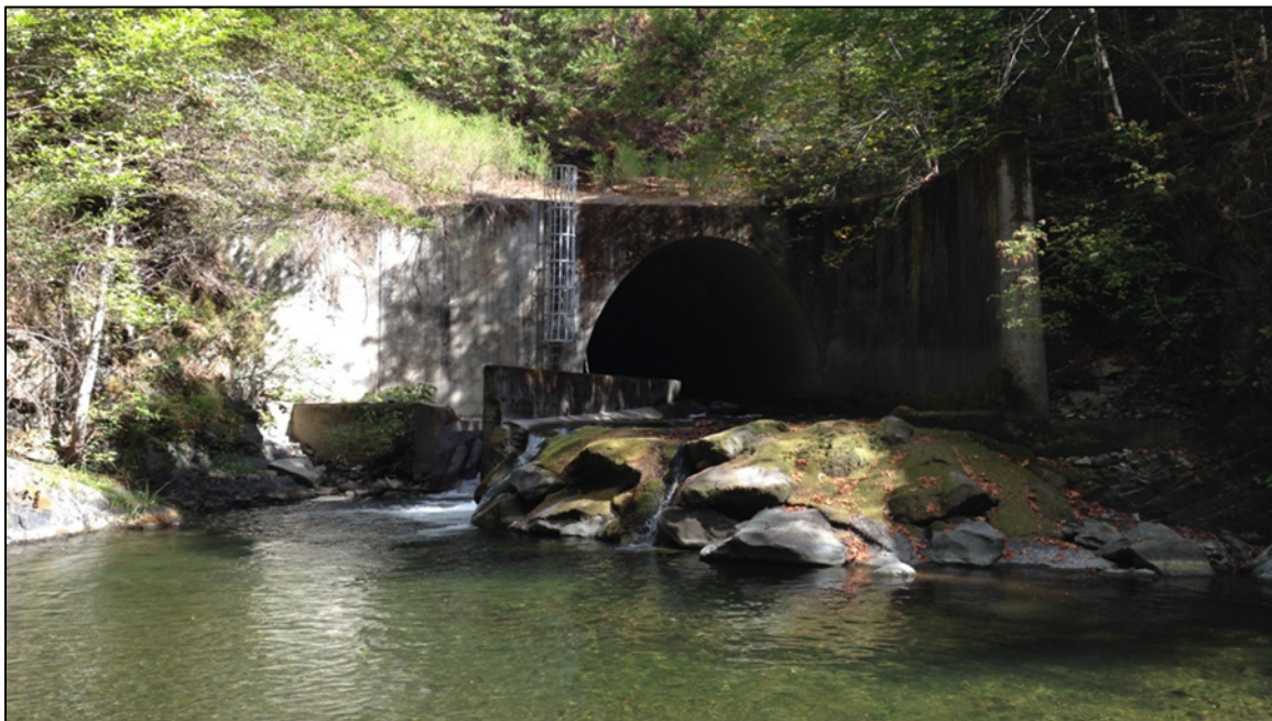
Figure 1. Pre-retrofit photo: culvert rock slope protection apron is perched above the water surface, Denil fish ladder for adult salmonid migration.
