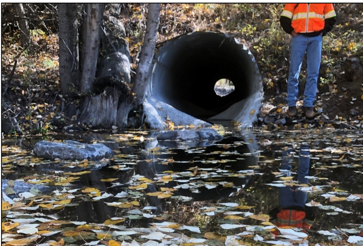
Figure 2. Marley Creek Culvert Outlet pre-project (top), with large perch creating barrier to upstream migrating fish and lamprey. After the project was completed, backwater conditions allow upstream fish migrations and rounded baffles were installed inside the culvert to add depth and reduce velocities.
