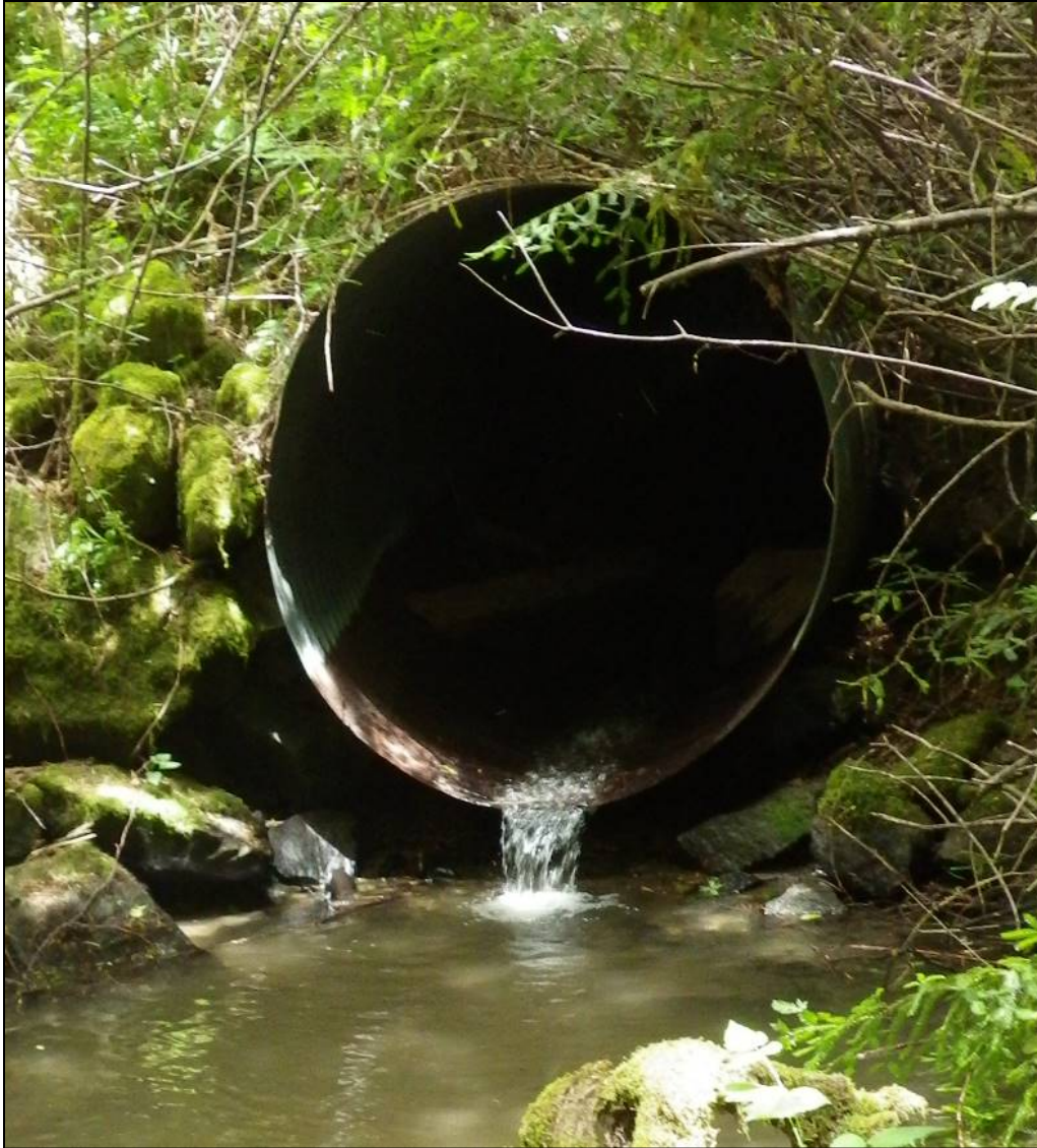
Figure 3. Example of perched and impassable road crossing, Strawberry Creek, Eel River basin, CA. Credit: Wiyot Tribe Natural Resources Department.
