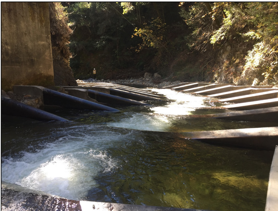
Figure 3. Post- project photo. Fishway with modified weir profiles installed downstream of the culvert. Rounded lamprey weir on left and squared salmonid weir on right.
