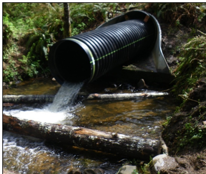
Figure 1. Coho Creek outlet prior to restoration. The perched, undersized and failing culvert was slip lined with a plastic pipe to prolong life.
