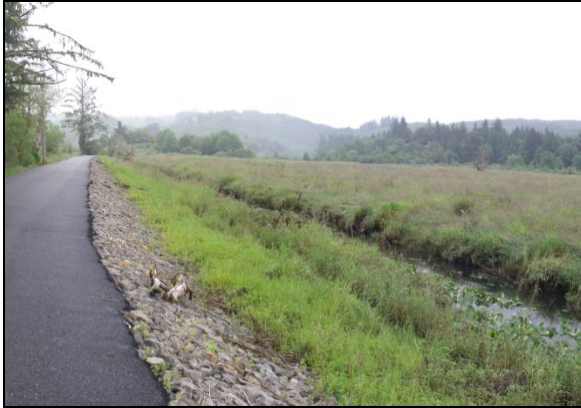
Previously established photo point (PP4E)
