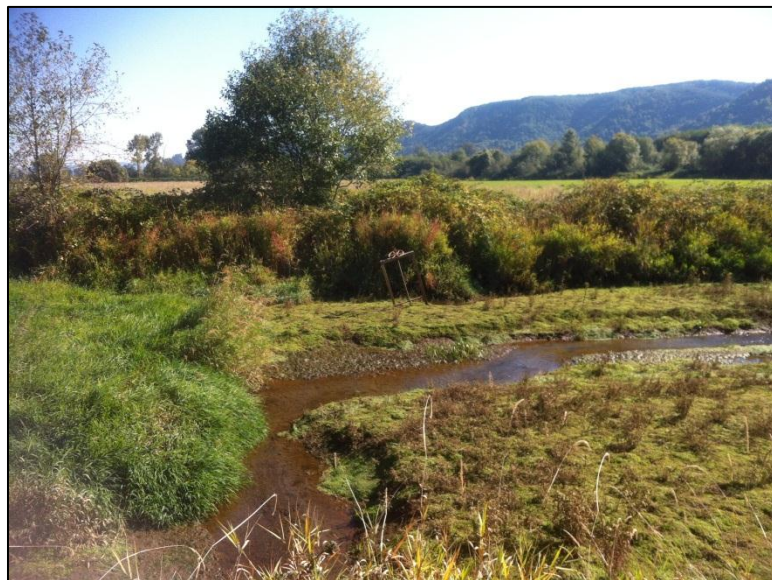
Figure 4 Looking at a tide gate on western side of dike from across the slough at low tide (Sept 2012)
