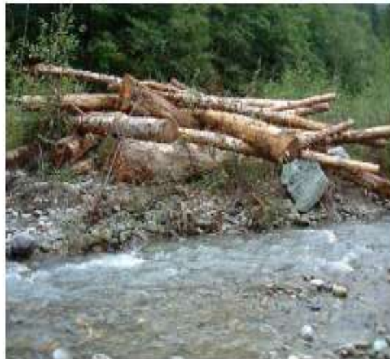
Large Wood and Log Jams Figure 3. LW placed on the floodplain will provide low velocity refuge during high flows. (Finney Creek, Skagit County, Washington).
