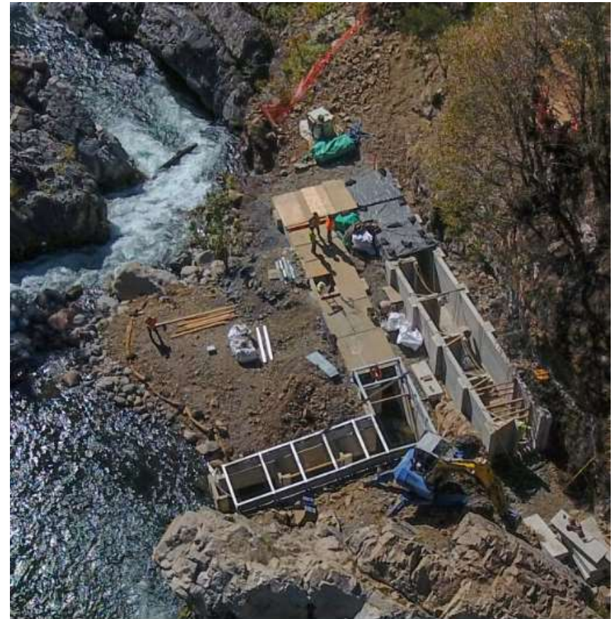
Deer Creek Fish Passage Improvement Photo Credit: NW Hydraulic Consultants 2020
