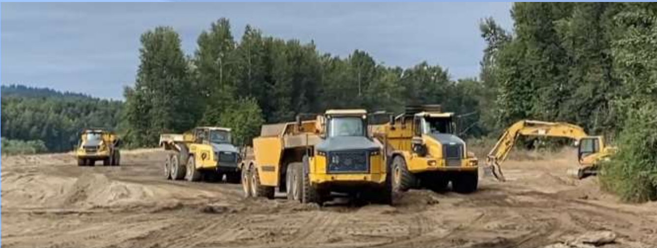
Lots of big equipment = compaction
