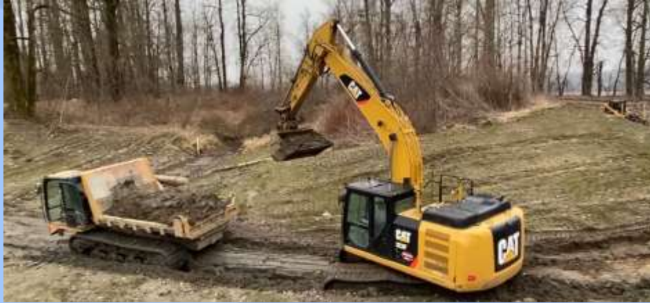
Main trail under construction during winter 2022
