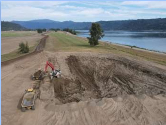
Sand & silt soils best for levee construction
