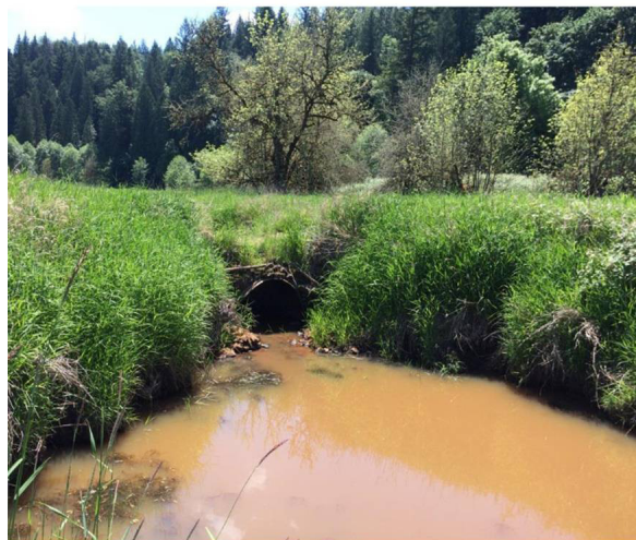
Site 43B culvert to be replaced with bridge.
